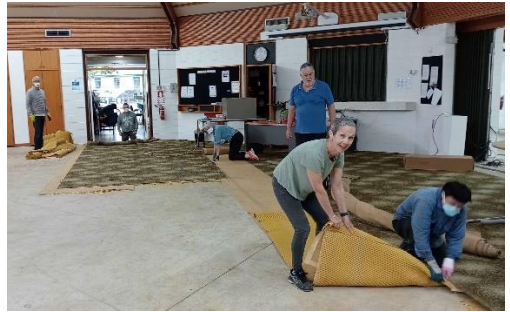
Below: Removing the old carpet
